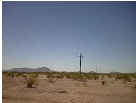
Site and transmission line looking north
